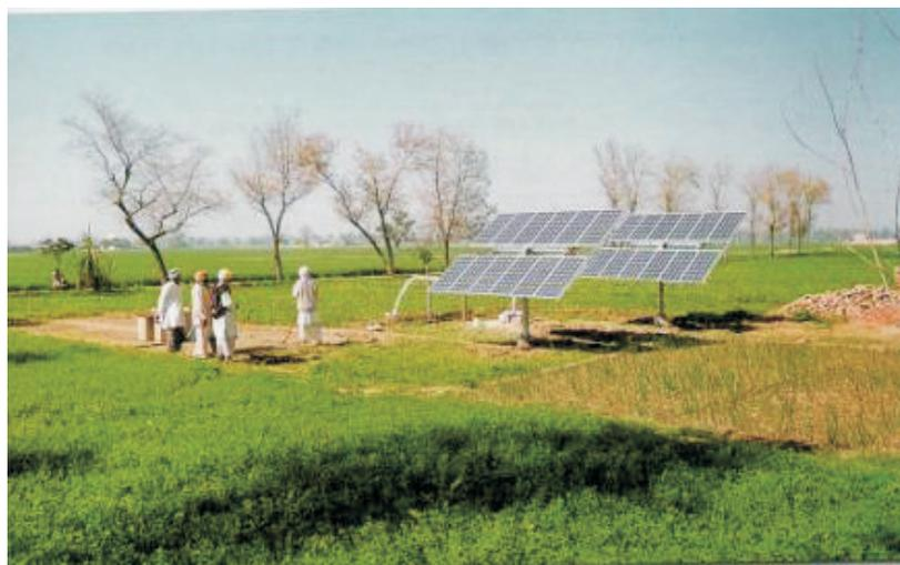
**Fig. 12.2** Photovoltaic Water Pumping
